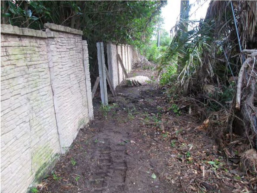
South side of South Perimeter Wall near west end
