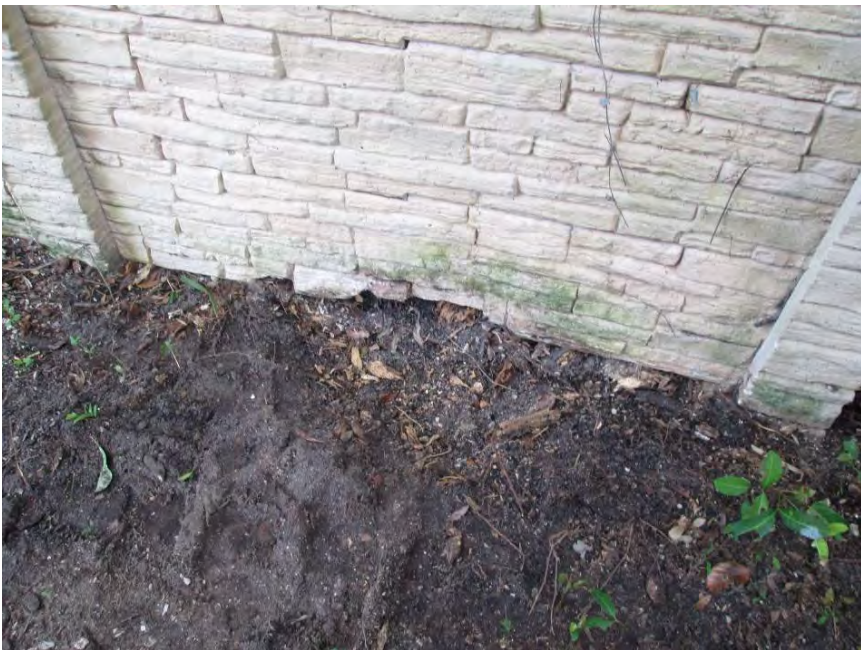
Stump along south wall near west end
