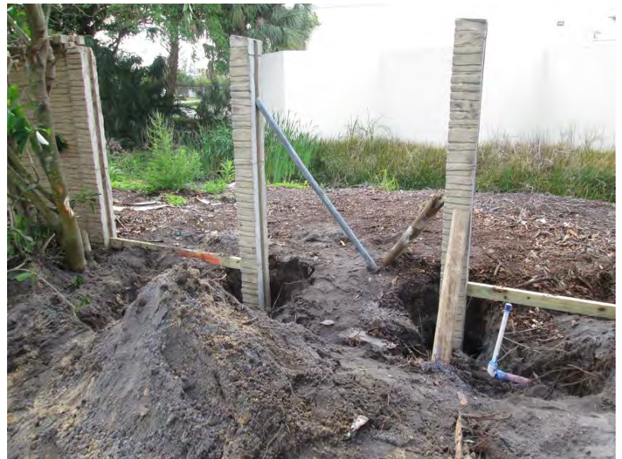
Post replacements for South Perimeter Wall near east end
